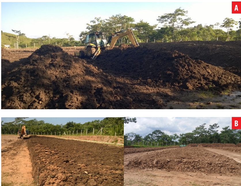
Figure 1. Bioremediation field assays. A) Windrows. B) Landfarming. Source: Authors.
